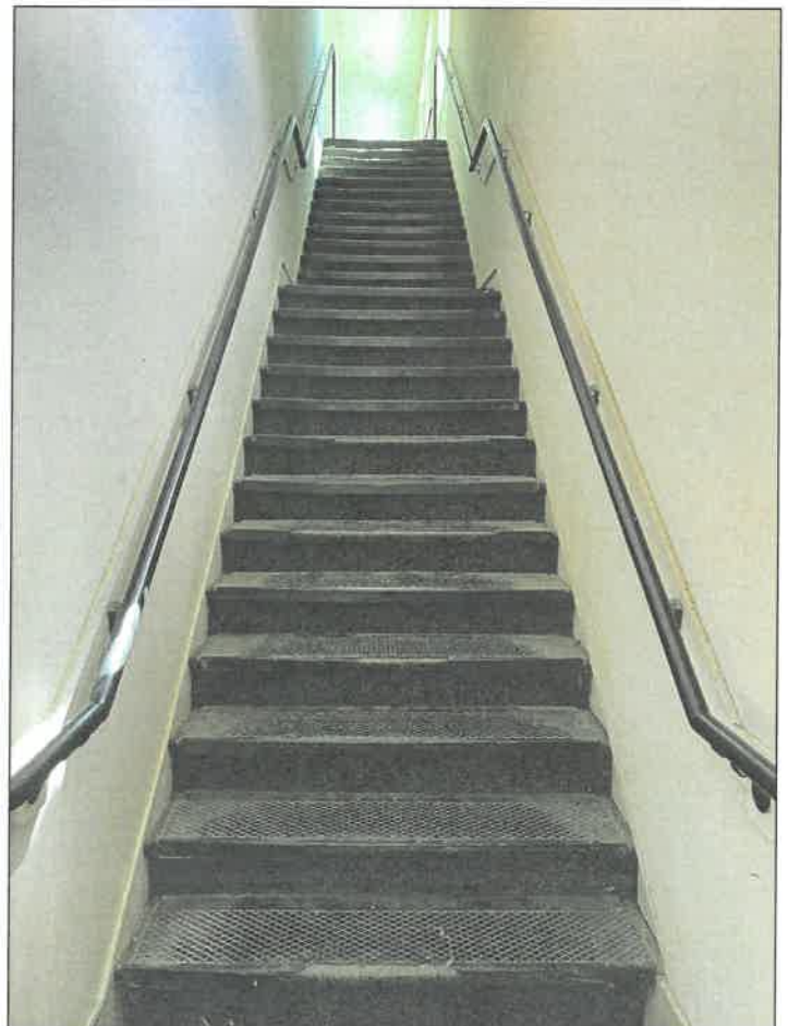
Stairway on west edge leads to the second floor
