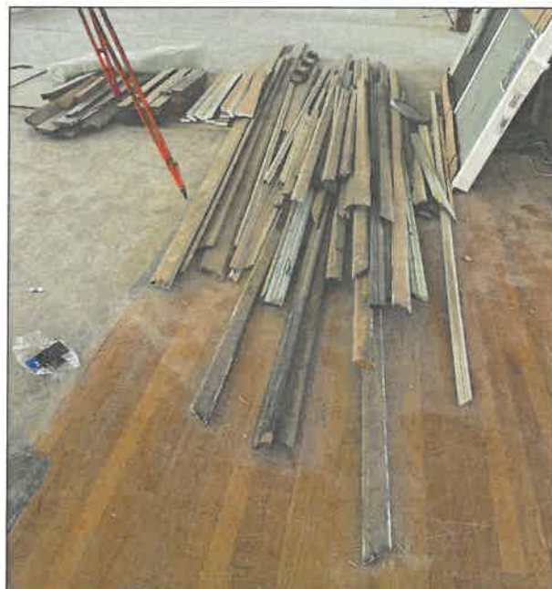
Trim and flooring have been salvaged during demolition and are ready for environmentally friendly reuse
