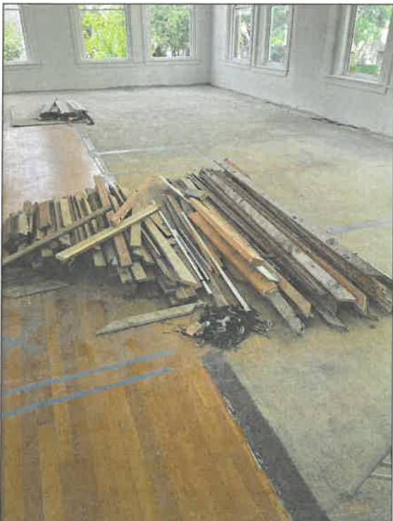
Trim and flooring have been salvaged during demolition and are ready for environmentally friendly reuse
