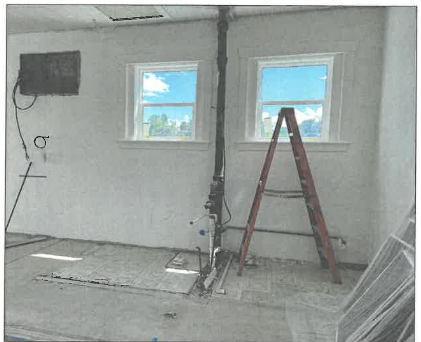
(Left) Most of the 27 windows have been replaced with Energy Star windows; (above) plumbing will be concentrated on the southern end
