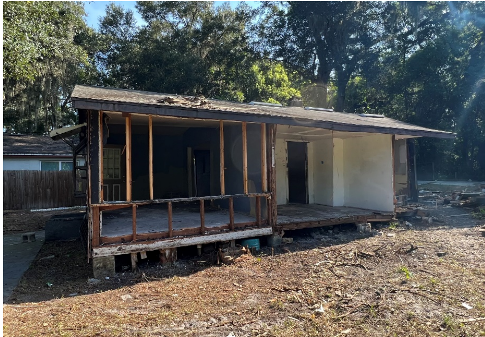
Figure 2: West View of Structure
