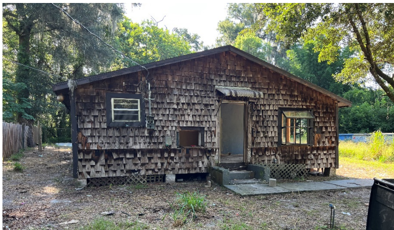
Figure 1: North View of Structure
