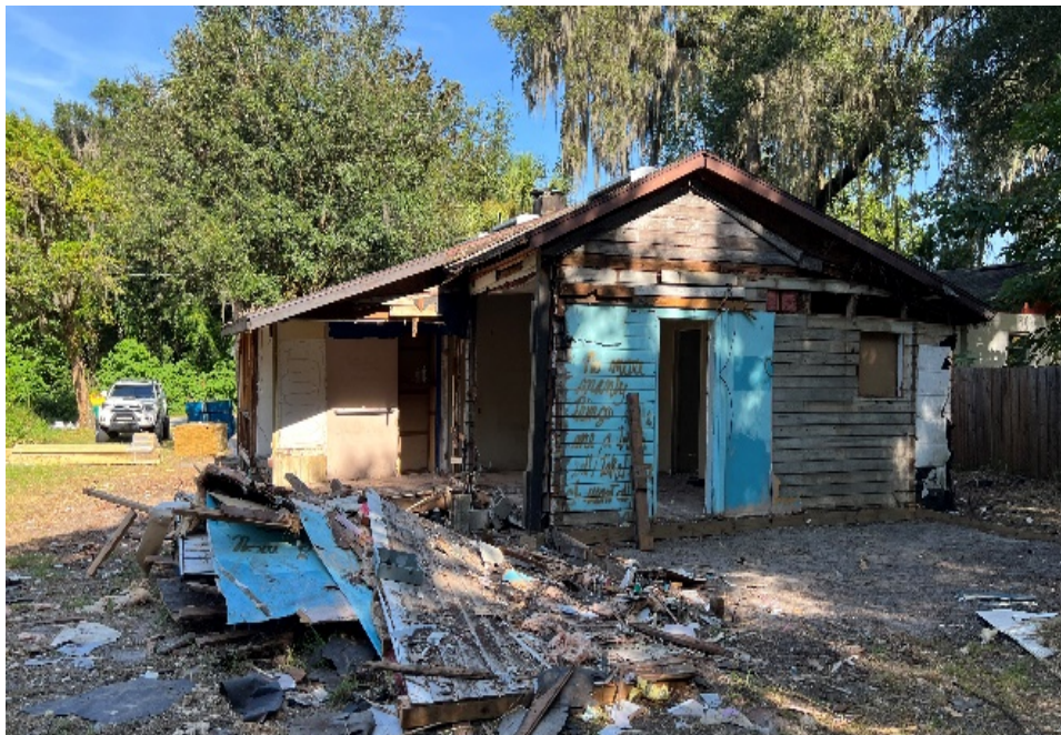
Figure 3: South View of Structure
