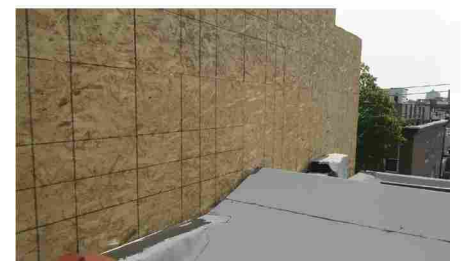
Figure 5. This interface between a rising wall and an existing roof will require careful detailing to exclude water. Any active chimney flues will also need to be extended above the new, higher roof line.
