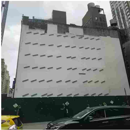
Figure 6. Former shared wall following demolition of existing building, with short lengths of steel channel attached to anchors bracing the masonry to floor structure at each level.
