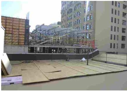
Figure 2. Inadequately secured sheets of plywood, intended for roof protection, can be dislodged by wind. This city's building code requires the plywood to be fastened over a layer of scaffold plank.
