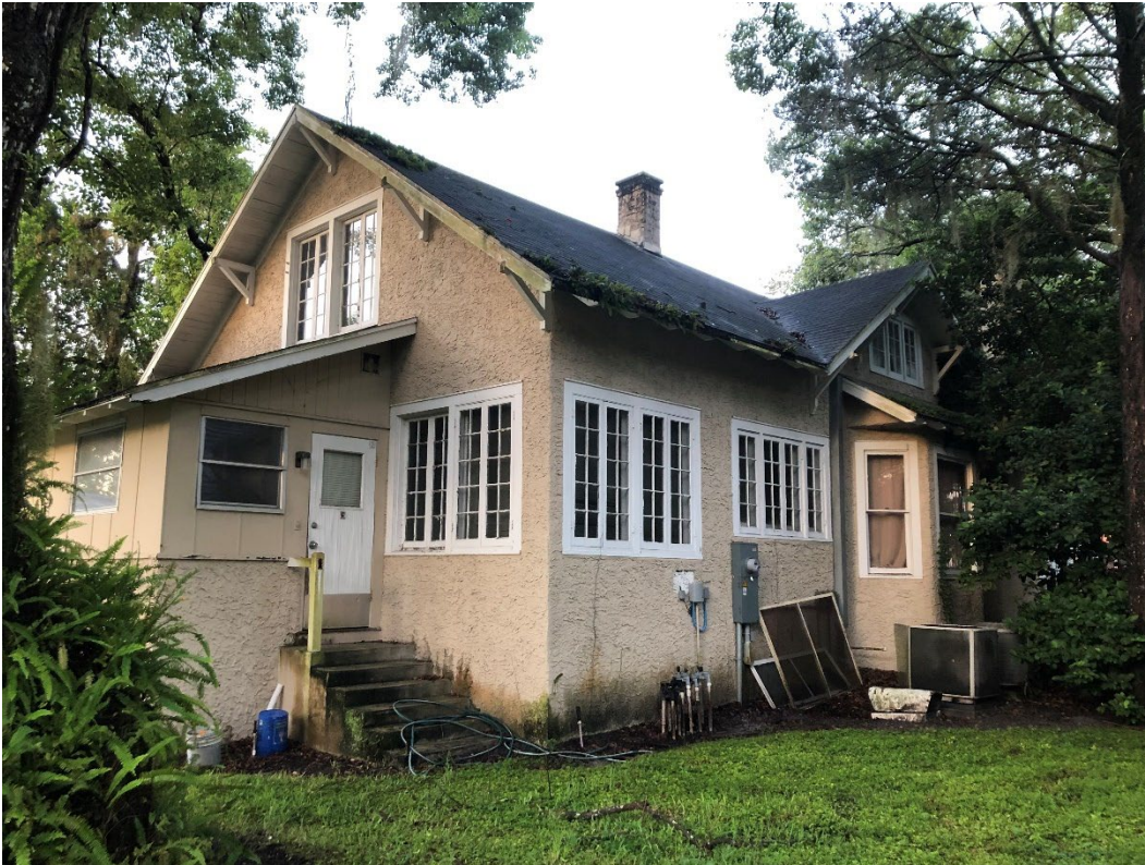
609 Bert Fish Drive, rear (east) and north elevations, facing southwest
