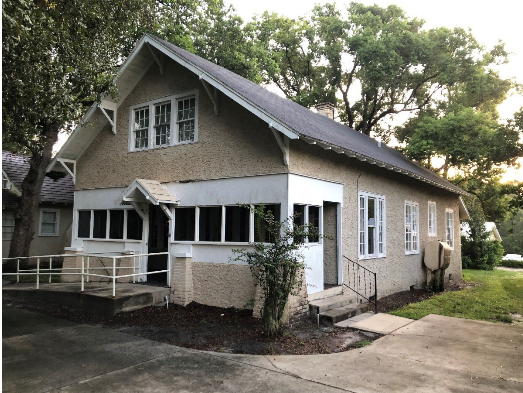
609 Bert Fish Drive, front (west) façade and south elevation, facing northeast
