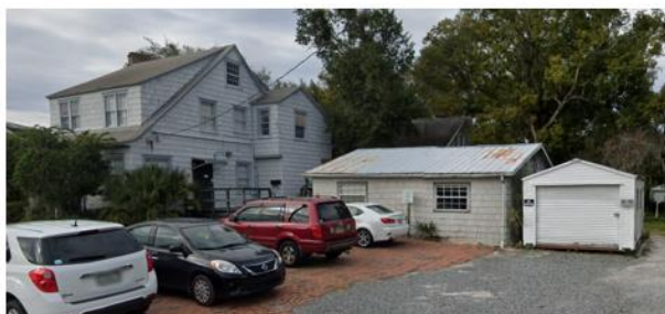
View looking toward the Northwest
