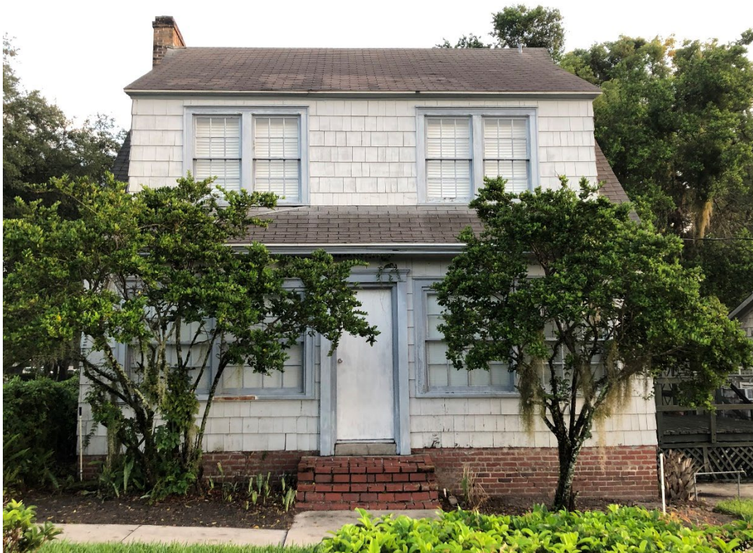
601 Bert Fish Drive, south elevation, facing north
