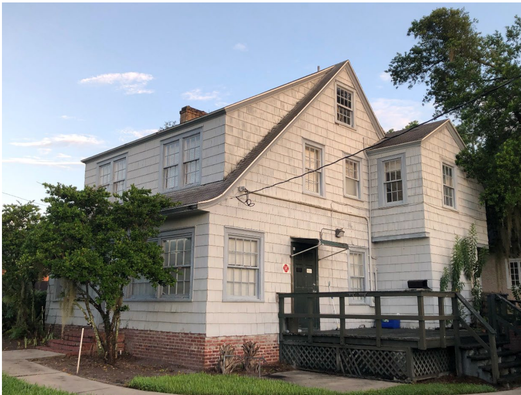
601 Bert Fish Drive, south and east (rear) elevations, facing northwest
