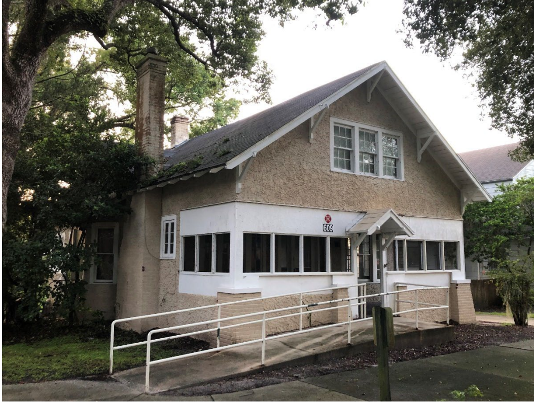
609 Bert Fish Drive, front (west) façade and north elevation, facing southeast
