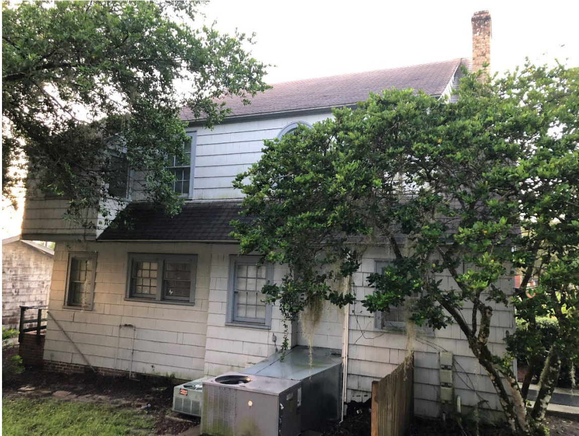
601 Bert Fish Drive, north elevation, facing south
