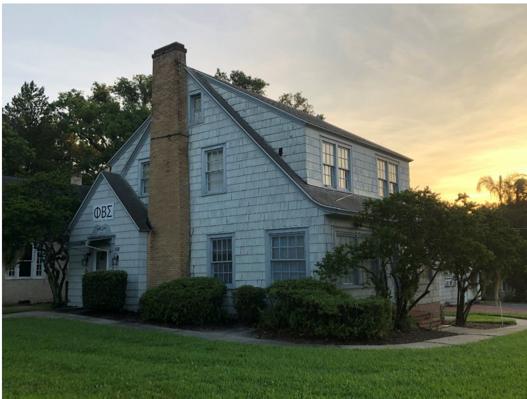
601 Bert Fish Drive, front (west) façade and south elevation, facing northeast
