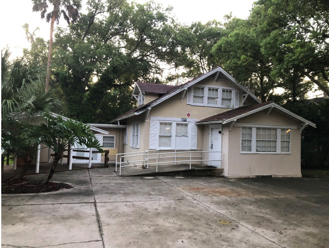
611 Bert Fish Drive, front (west) façade and north elevation, facing southeast
