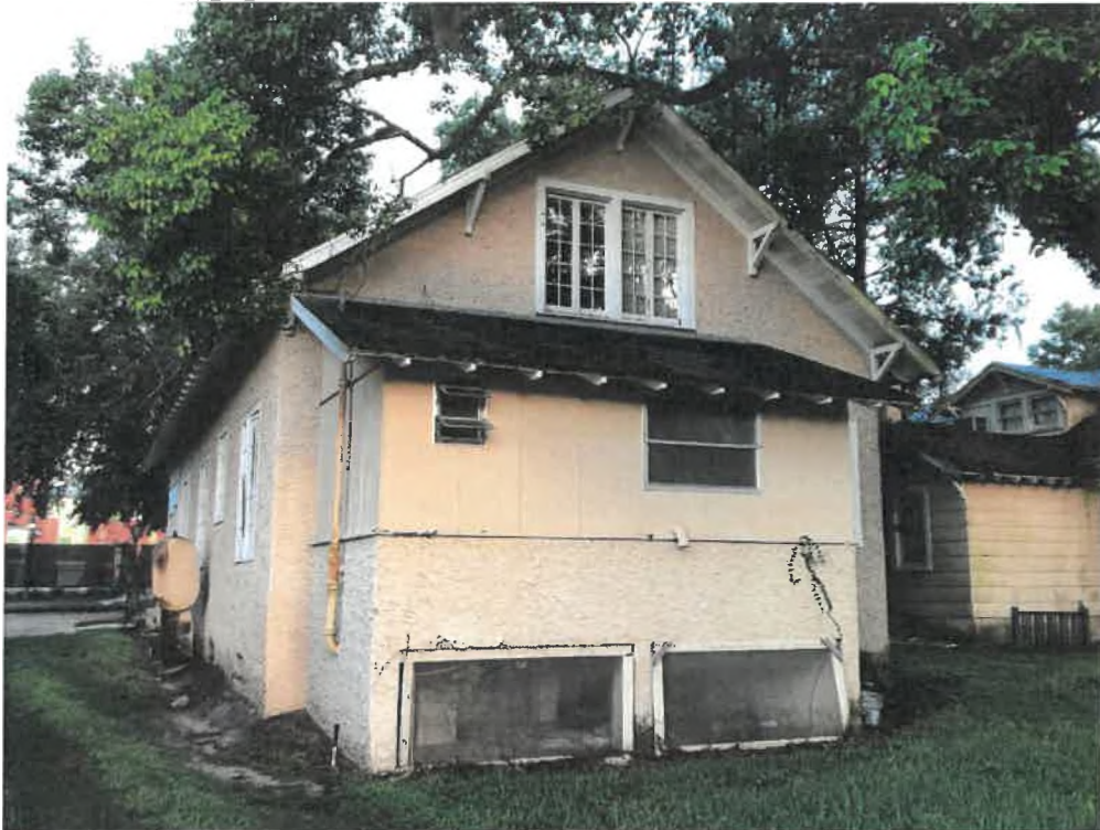
609 Bert Fish Drive, rear (east) and south elevations, facing northwest
