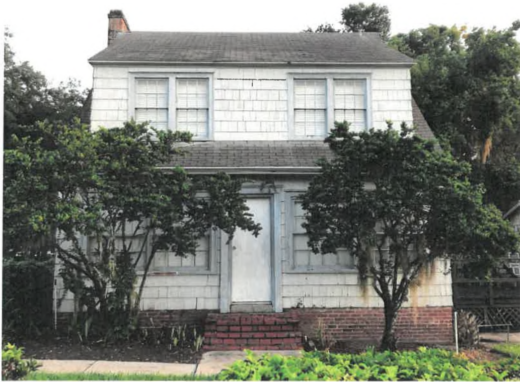
601 Bert Fish Drive, south elevation, facing north
