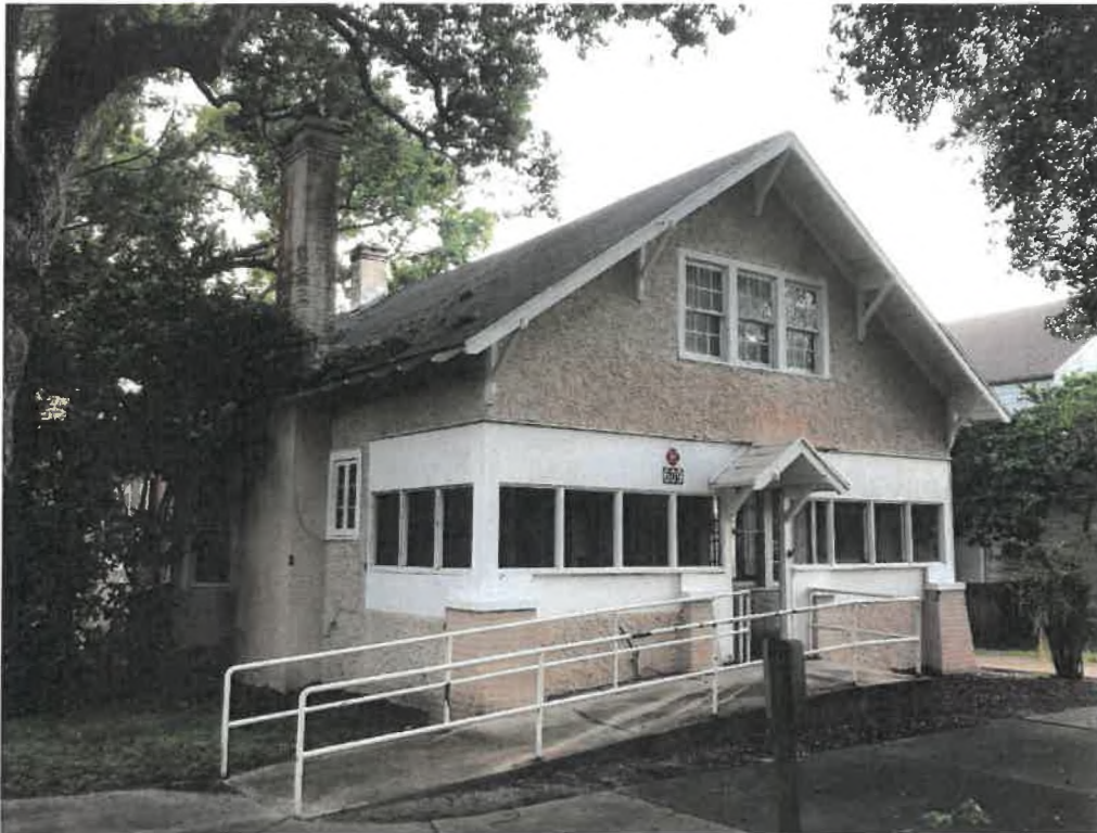
609 Bert Fish Drive, front (west) façade and north elevation, facing southeast
