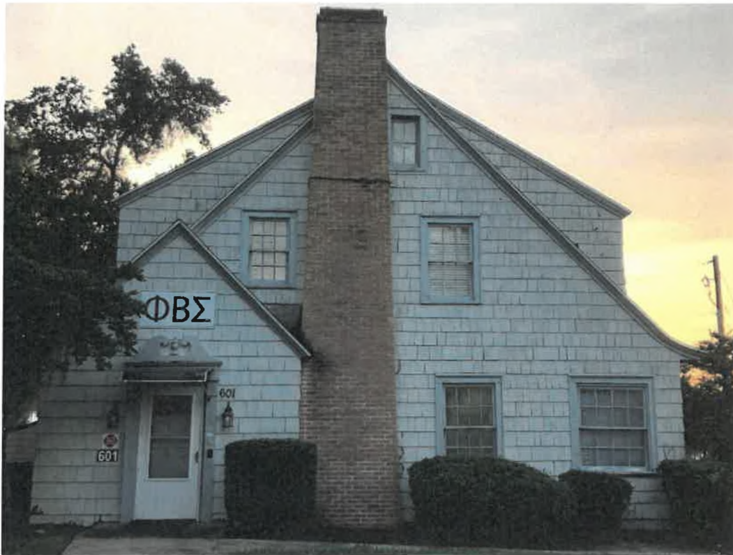
601 Bert Fish Drive, front (west) façade, facing east
