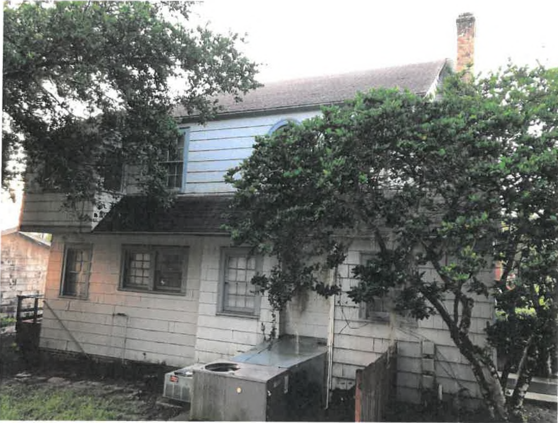
601 Bert Fish Drive, north elevation, facing south
