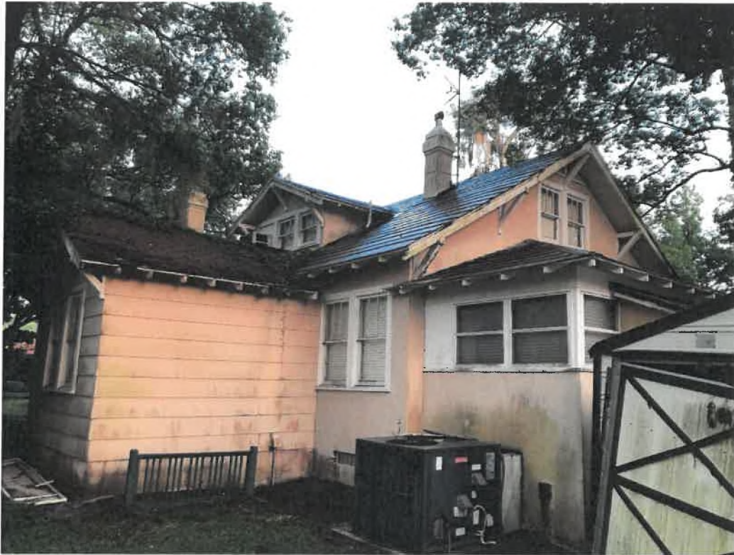
611 Bert Fish Drive, rear (east) and south elevations, facing northwest
