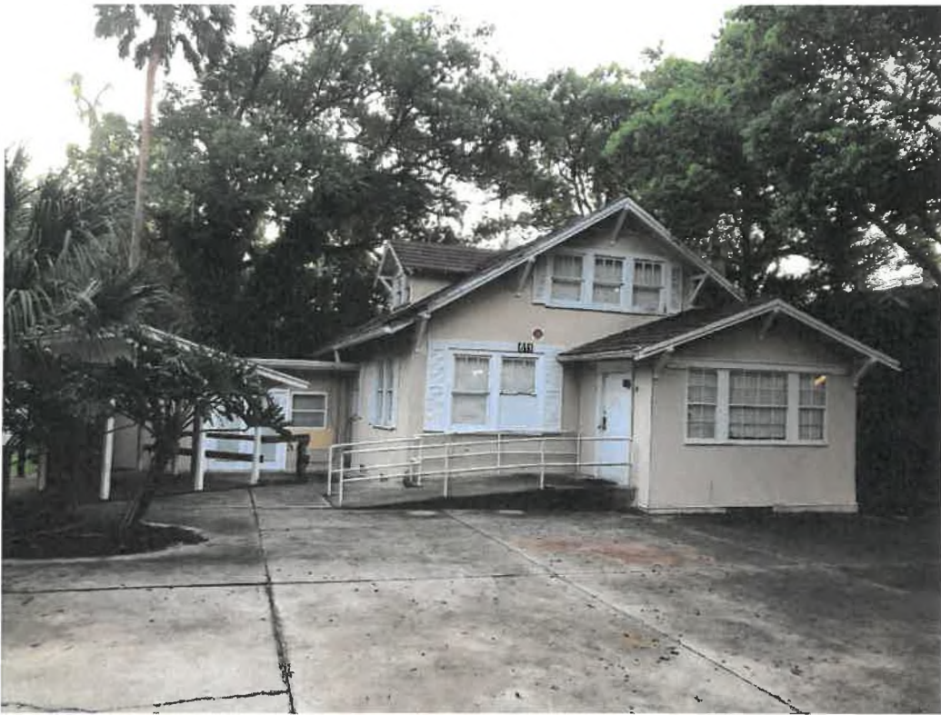
611 Bert Fish Drive, front (west) façade and north elevation, facing southeast
