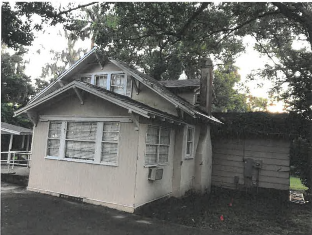
611 Bert Fish Drive, front (west) façade and south elevation, facing northeast
