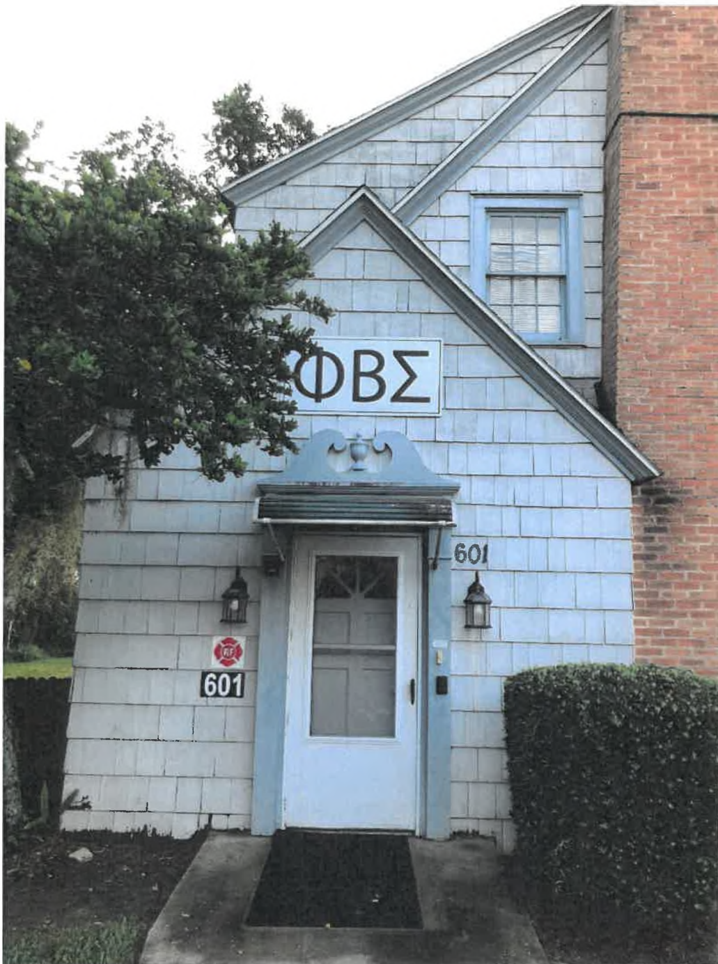
601 Bert Fish Drive, detail of front (west) entrance, facing east
