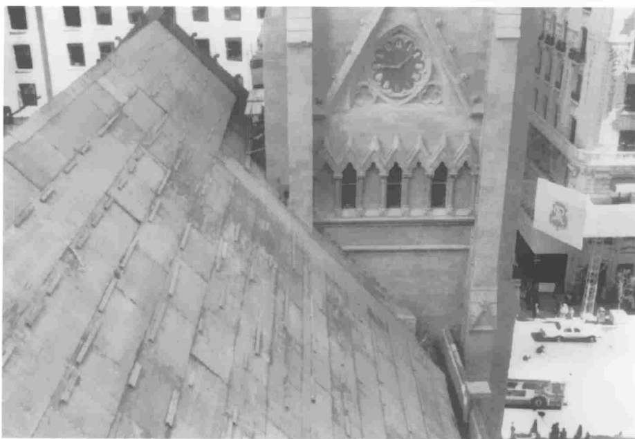
Figure 4. Dropped equipment, tools, and materials all present risks when new construction rises above neighboring historic structures. In this case, the historic slate roof was completely covered with sheets of exterior grade plywood. Photo: National Park Service files.
