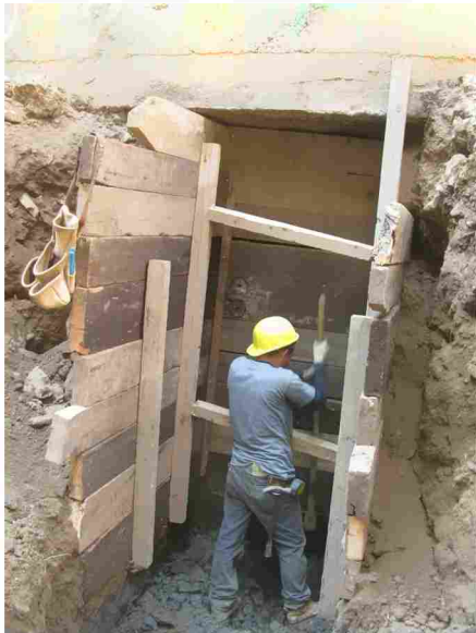
Figure 4. Timber sheeting at underpinning approach pit with adjacent areas improperly excavated alongside the existing foundation, increasing the risk of soil movement.
