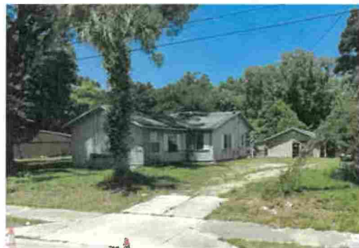
House and garage/carport
