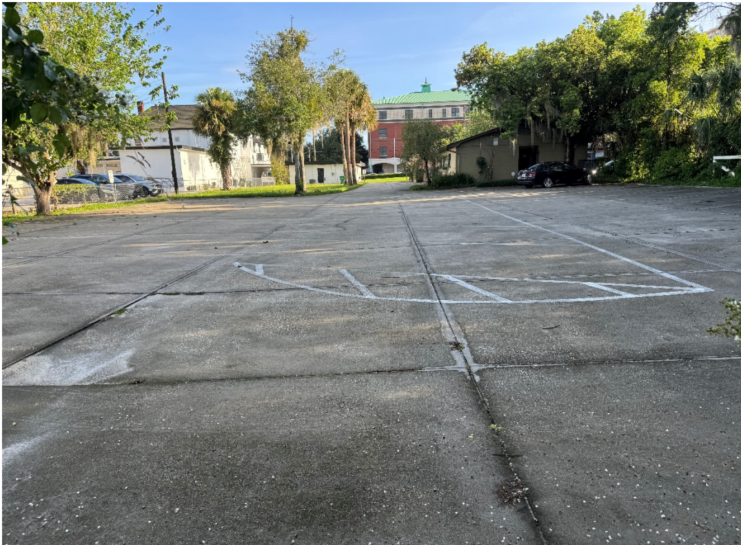
SUBJECT PROPERTY EXISTING PARKING LOT LOOKING NORTH
