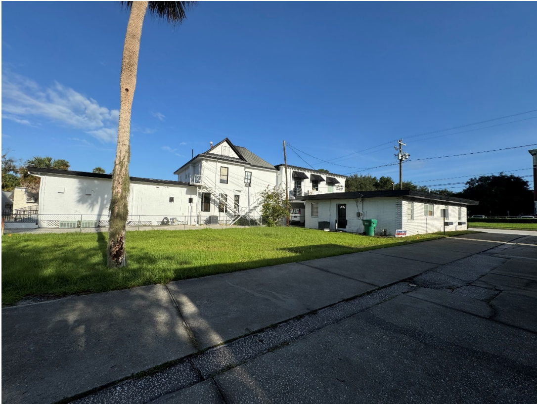
SUBJECT PROPERTY LOOKING NORTHWEST
