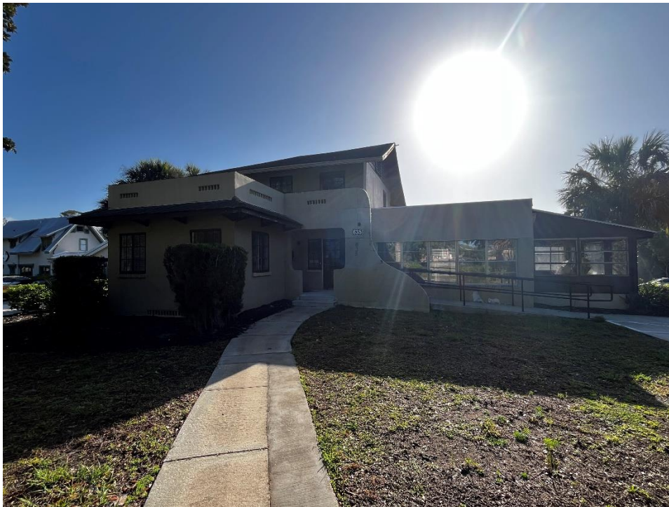
West elevation facing Bert Fish Drive
