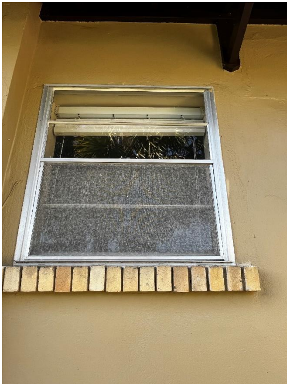
Deteriorated aluminum windows
