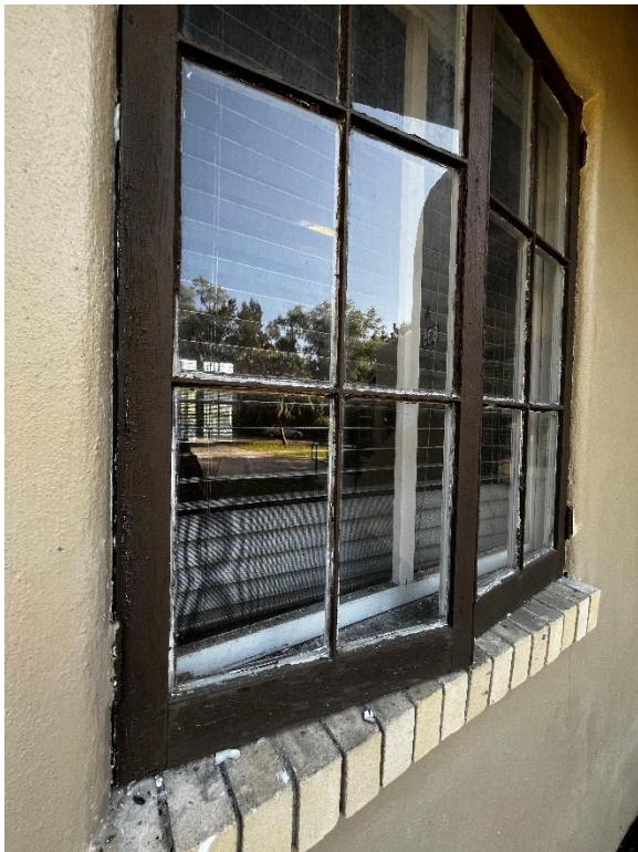
Deteriorated wood windows
