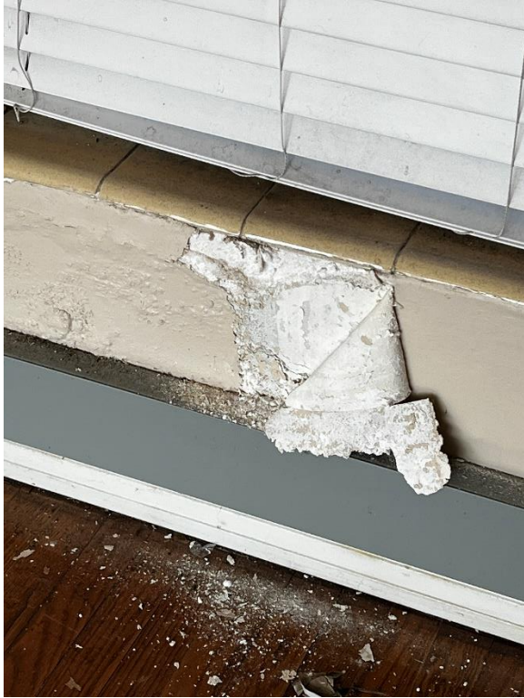
Interior water damage under aluminum windows
