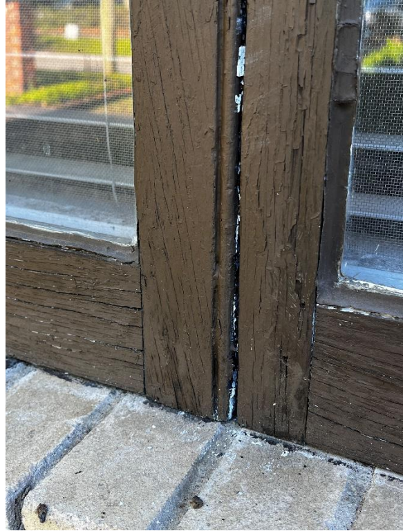
Deteriorated wood windows
