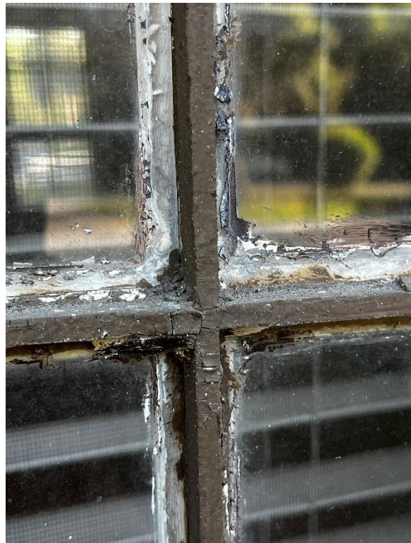
Deteriorated wood windows
