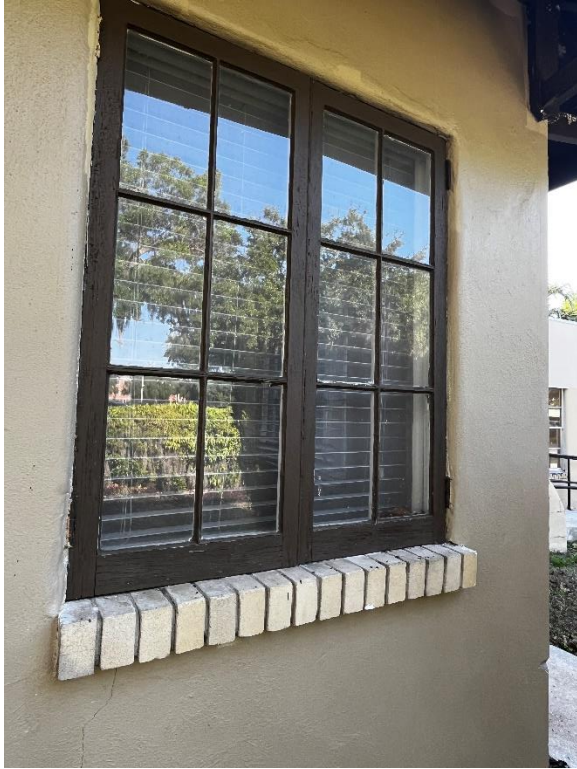
Deteriorated wood windows
