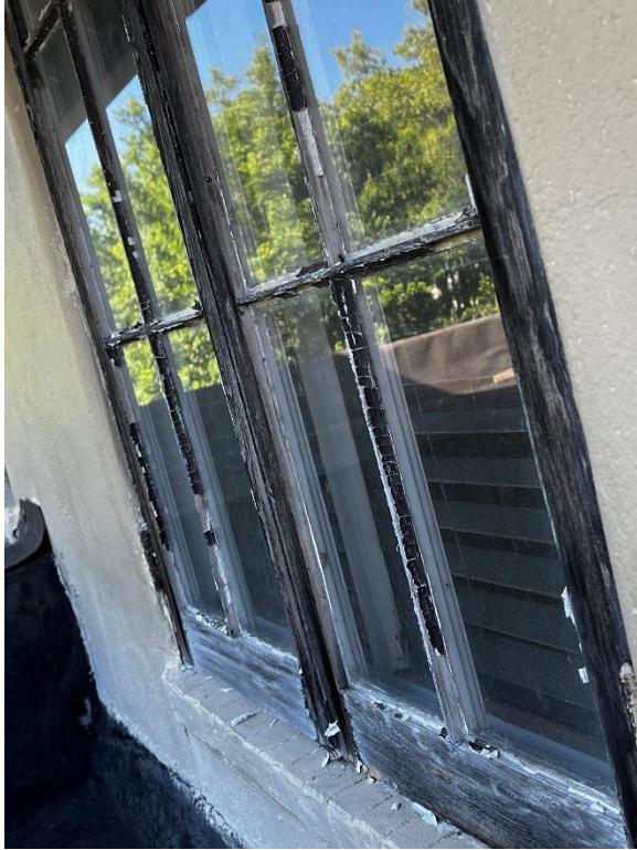
Deteriorated wood windows
