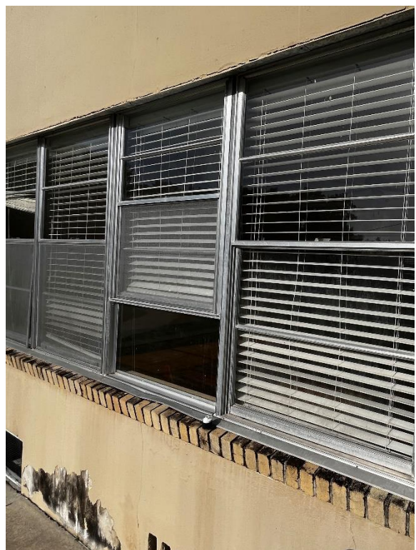
Deteriorated aluminum windows
