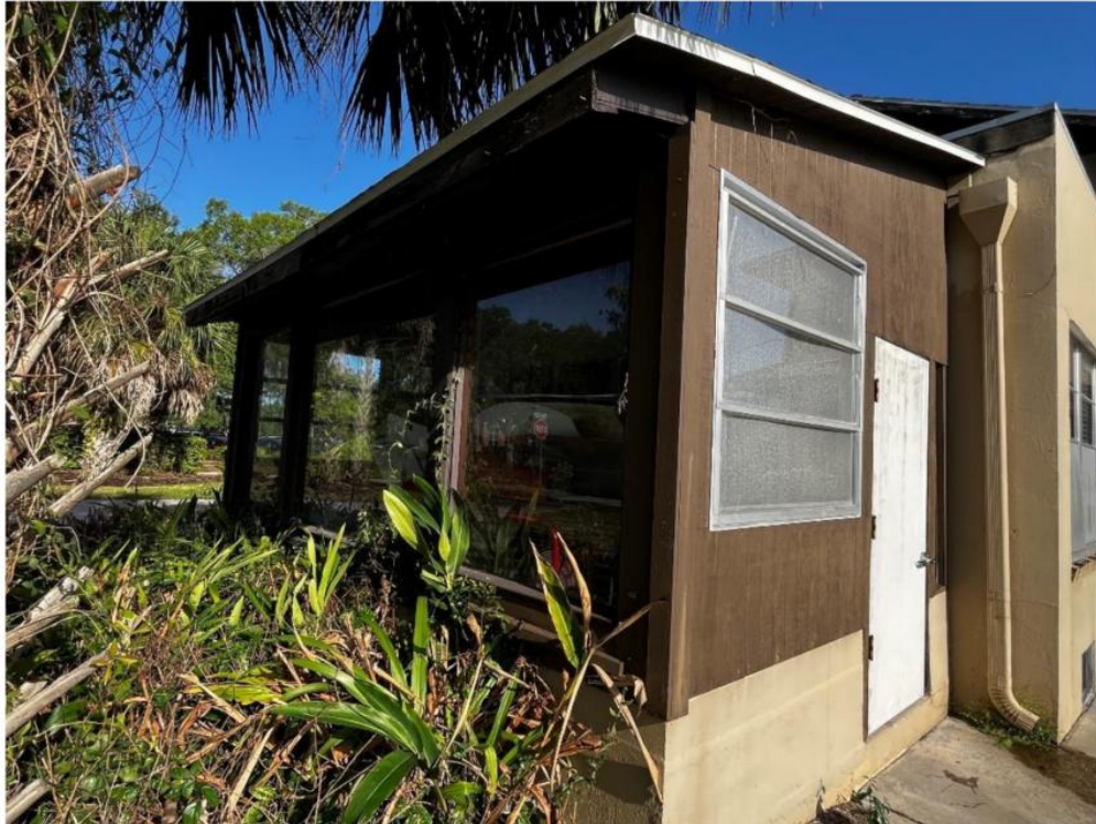
Lean-to addition, former greenhouse, facing south
