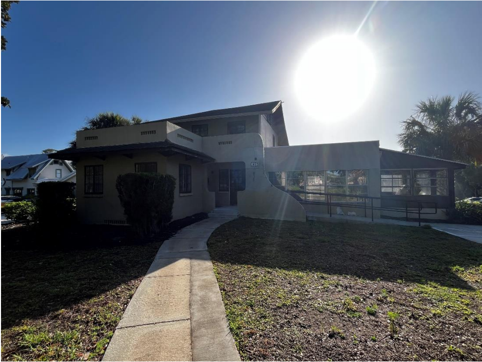
West elevation facing Bert Fish Drive
