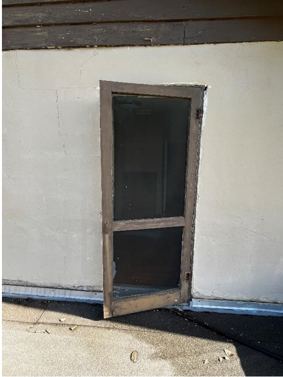
Screen door at roof access
