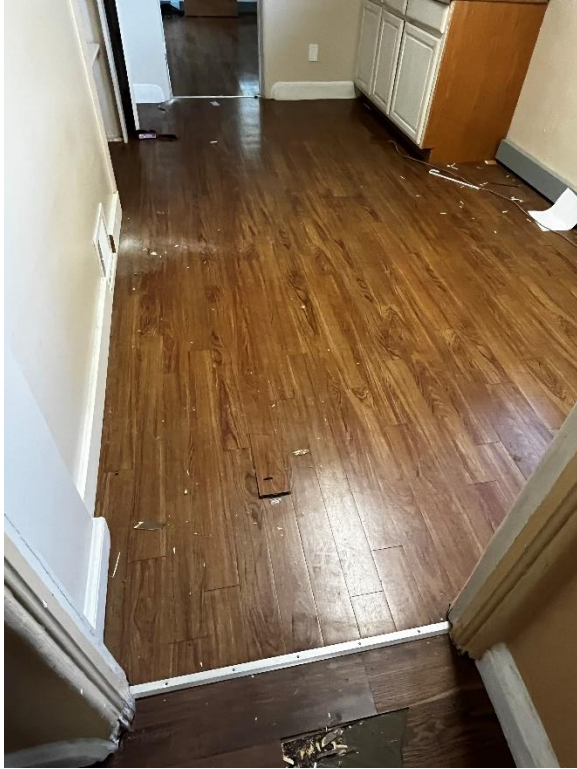
Vinyl plank flooring
