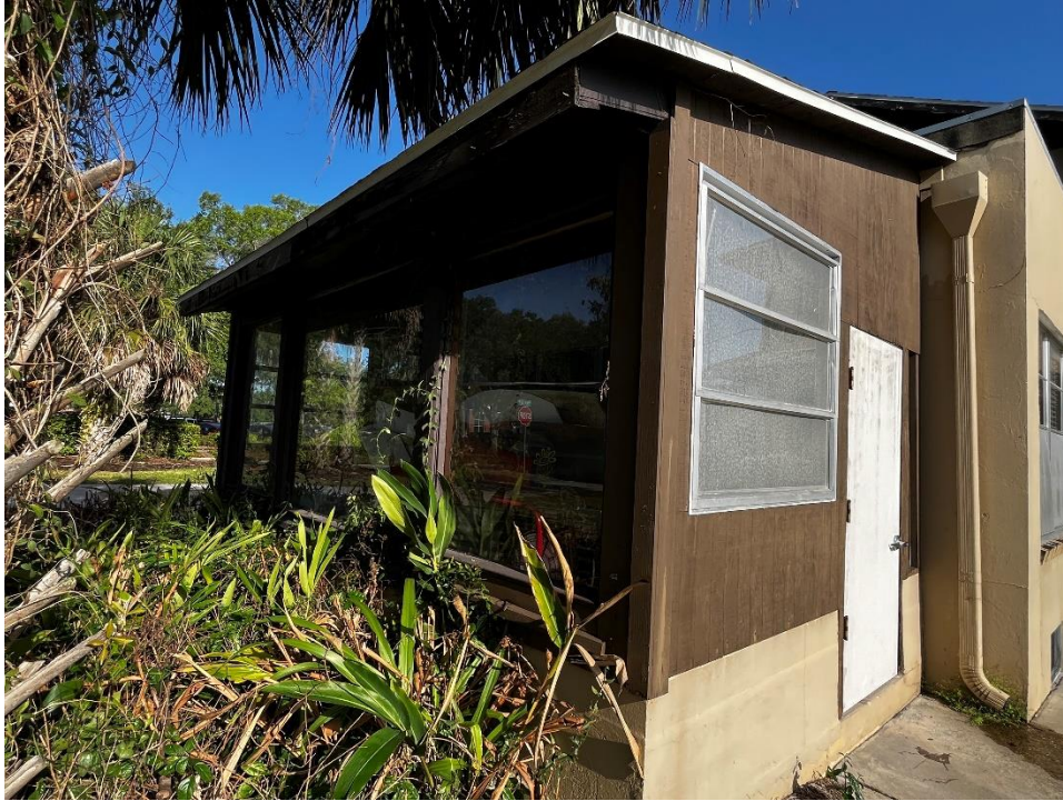
Lean-to addition, former greenhouse, facing south
