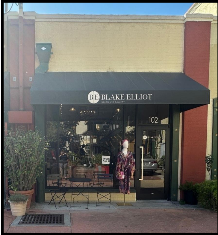
FIGURE 1 102 Artisan Alley Glass Storefront doors/windows
