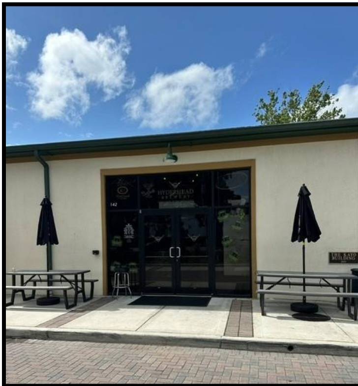
FIGURE 2 142 W Georgia Ave Glass Storefront doors/windows
