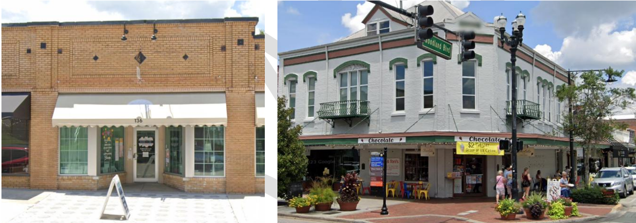
L: Storefronts with recessed entry; R: Storefront with corner entry
