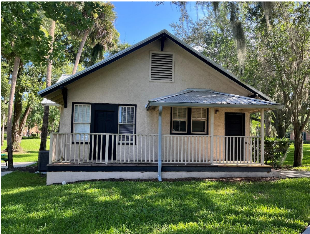
207-1/2 E Michigan, south (rear) elevation
