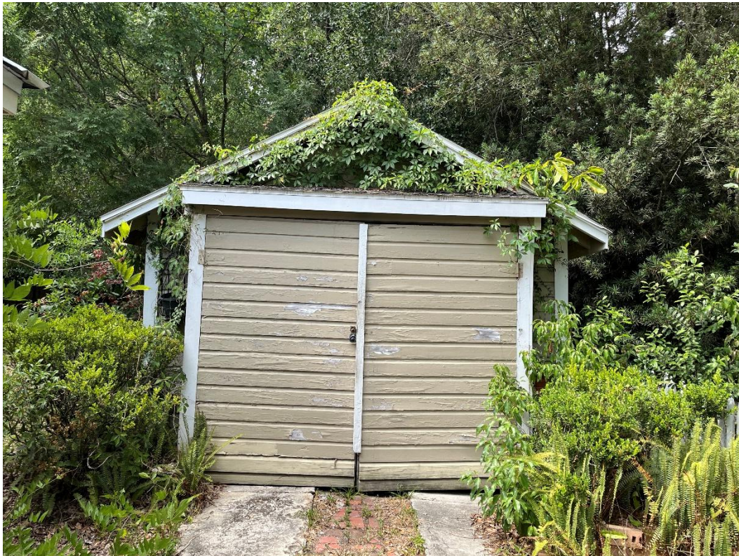
209 E University, south elevation of detached garage
