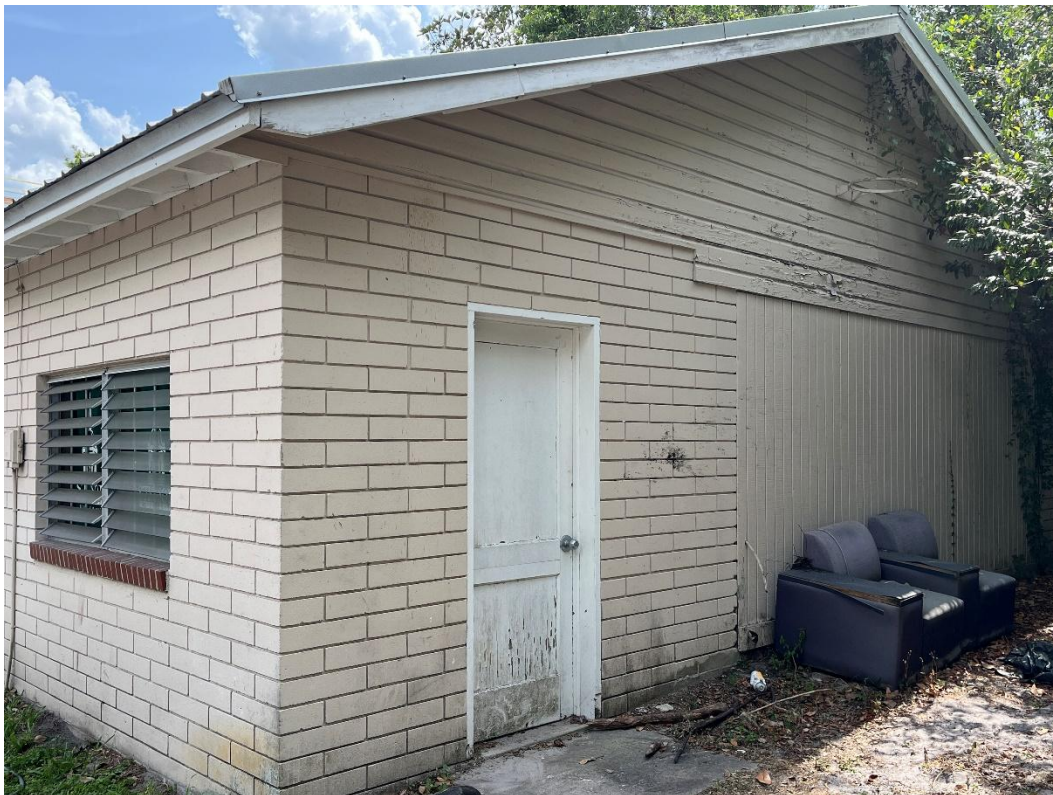
205 E University, north and east elevation of detached garage
