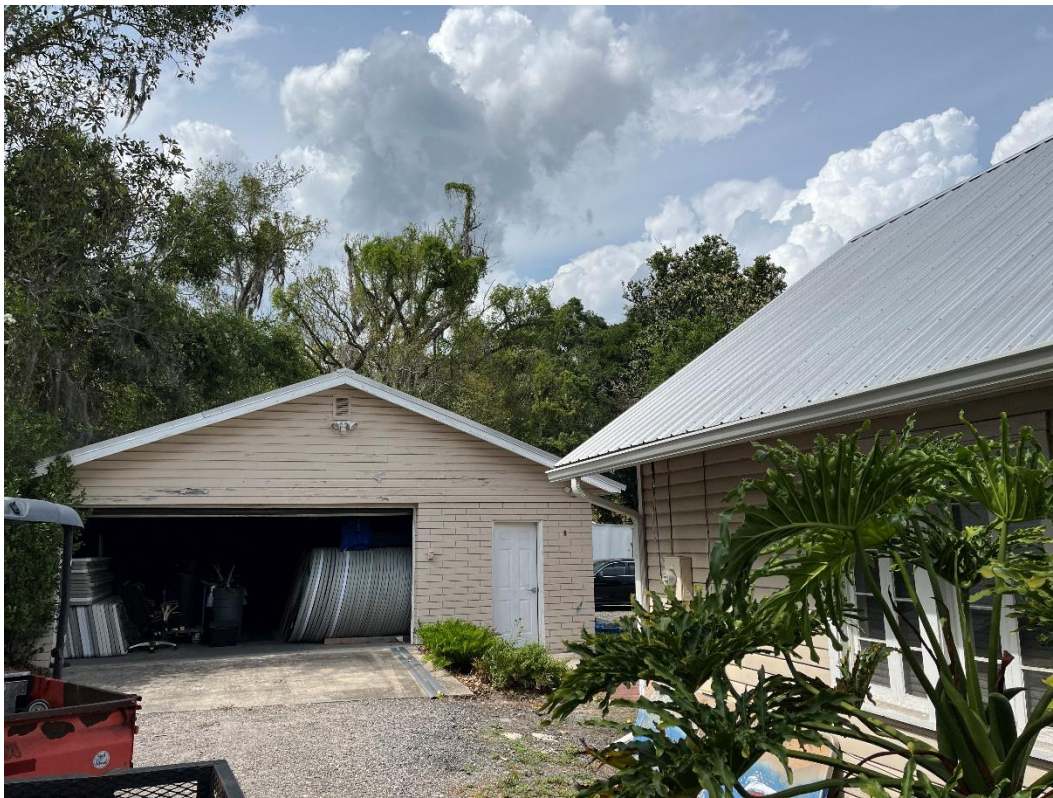
205 E University, west elevation, and south elevation of detached garage
