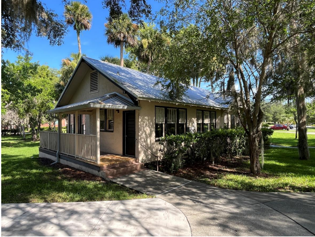
207-1/2 E Michigan, south (rear) and east elevations, facing northwest
