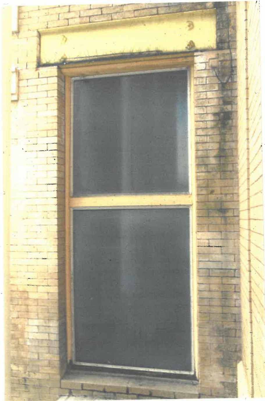
NORTH WALL WINDOW LOOKING SOUTH
