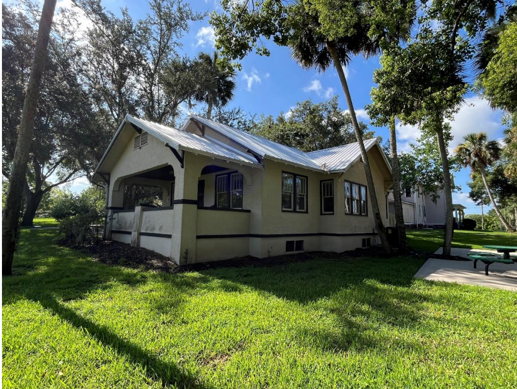
207-1/2 E Michigan, north and west elevations, facing southeast
