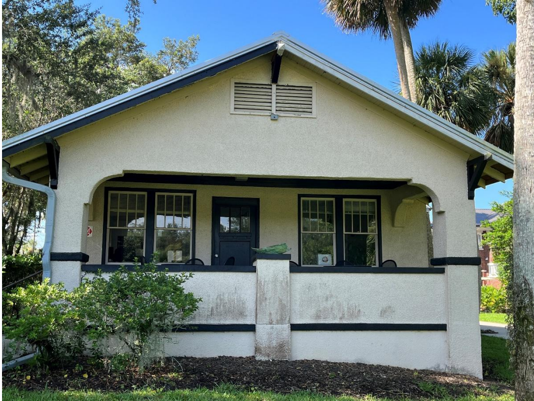
207-1/2 E Michigan, front (north) elevation
