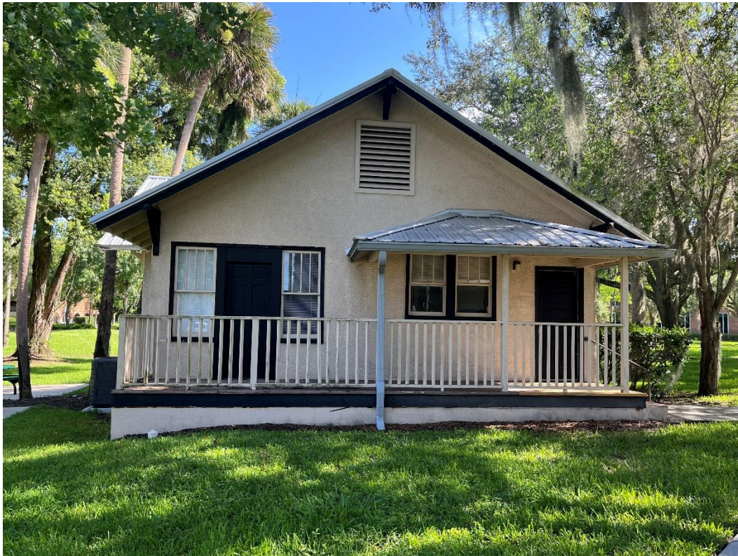
207-1/2 E Michigan, south (rear) elevation
