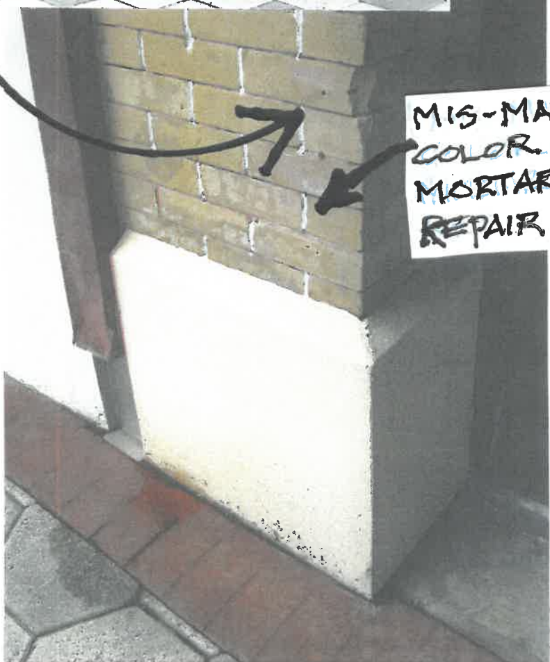
PHOTO DETAILS OF COLUMN DETERIORATION
