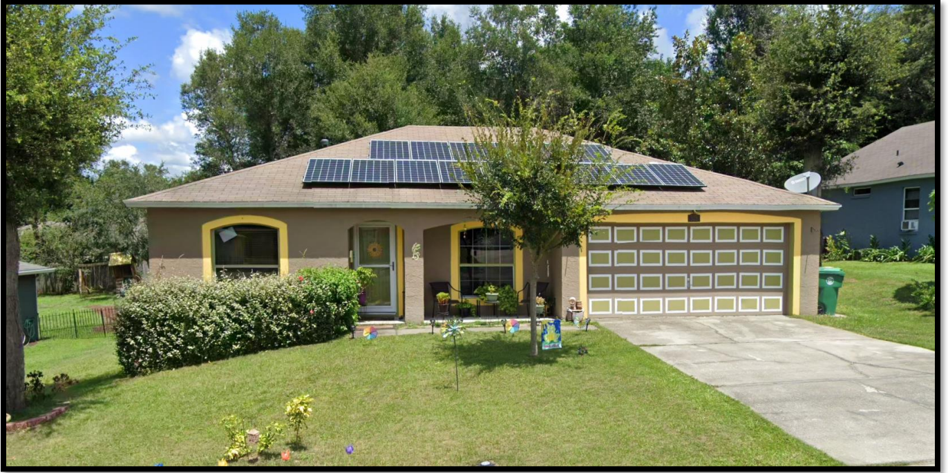
515 John Thomas Avenue - Previous Elevations (before renovation)
