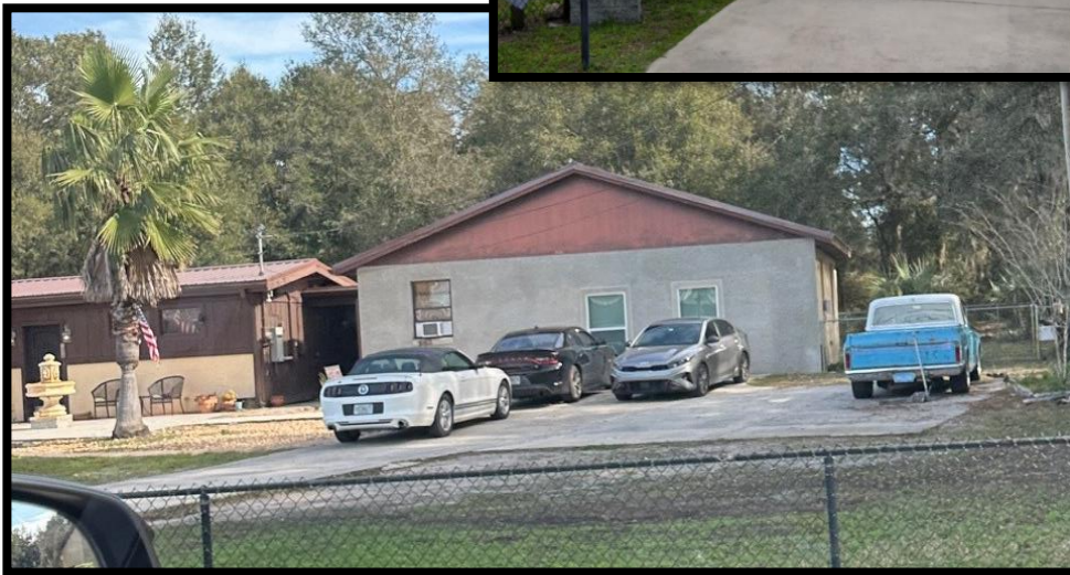
1335 Aquarius Avenue Previous Elevations (After renovation)
