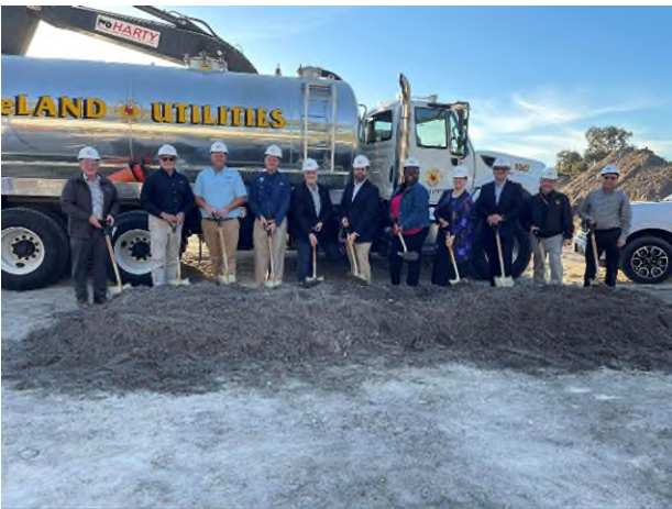
DeLand Water Treatment Site
